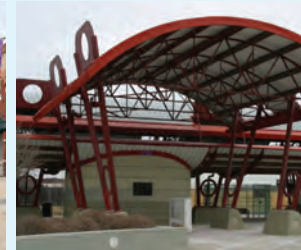
Northwest Transportation Center
